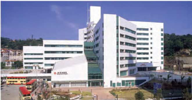
Tseung Kwan O Hospital, Hong Kong, China
