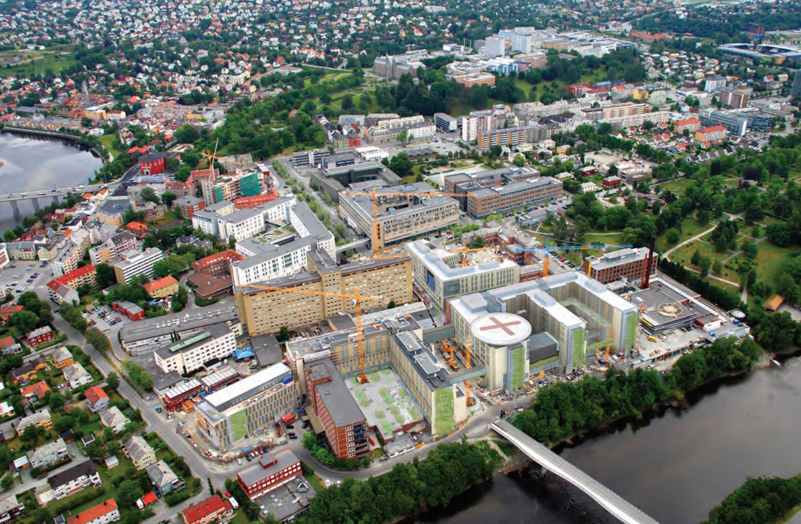
Figure 1: Sophisticated hospitals need sophisticated IT resources to achieve optimum efficiency. St Olav's Hospital in Trondheim, Norway – a 'digital hospital' – features automated, coordinated operating systems
