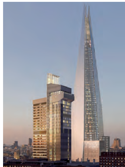
Figure 3: New superinsulated cladding for Guy's Hospital tower, London, devised by Penoyre & Prasad and Arup, will reduce energy use by 15-20%
