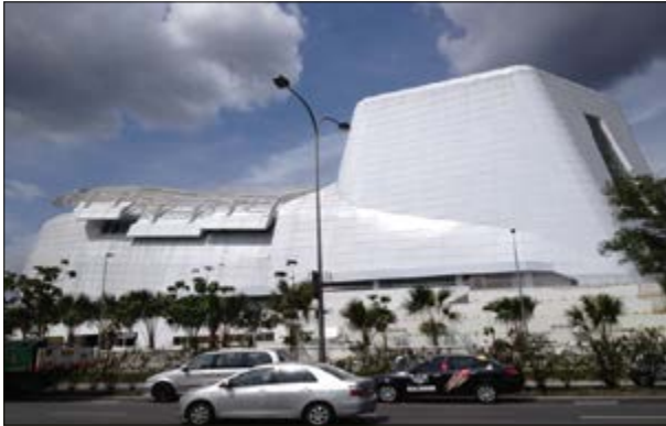
Calvary Convention center; Malaysia – The operable roof for mixed mode cooling.
