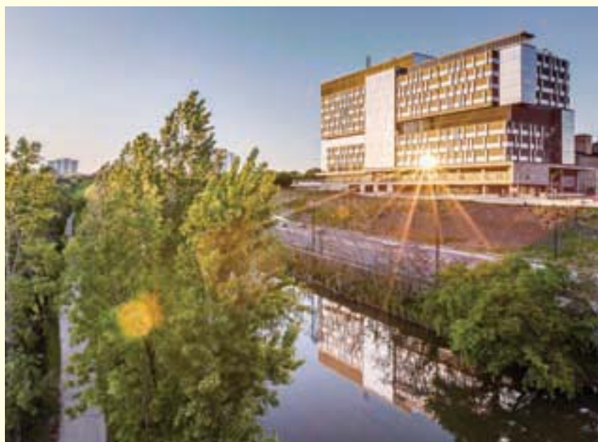
Figure 1: Stantec and KPMB's Bridgepoint Hospital in Toronto, subject of a post-occupancy evaluation
