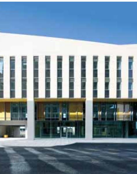
Glazed brickwork and matching mortar creates a monolithic appearance
