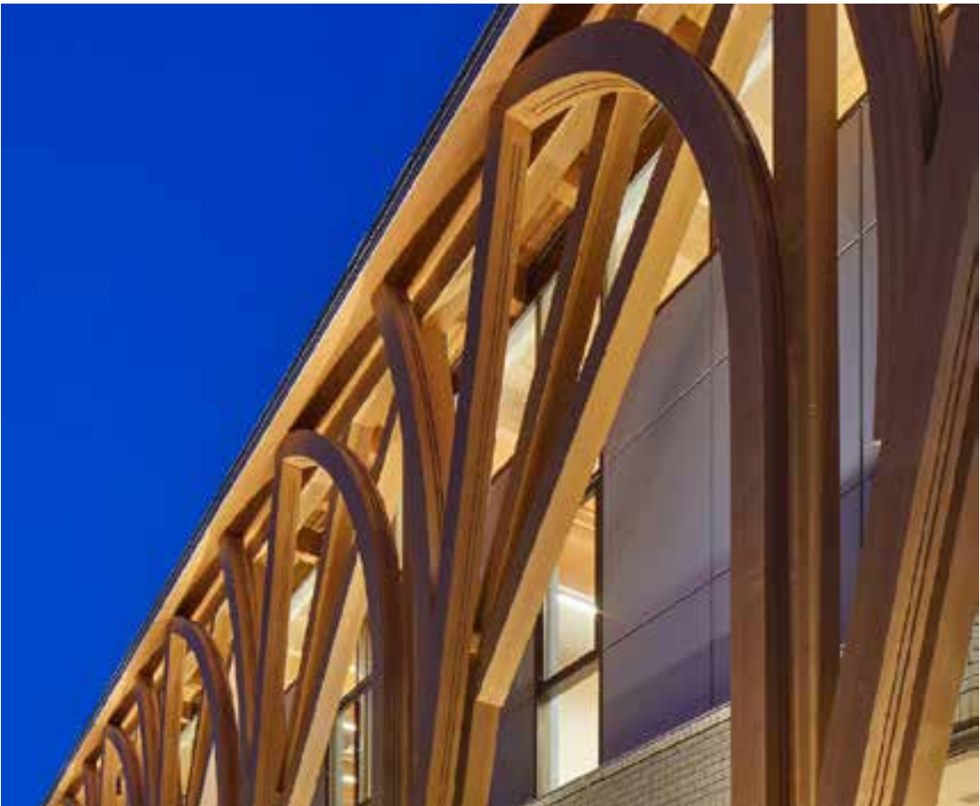
Consonance and dissonance: the TMS Upper School's middle school wing exoskeleton timber structure, Farrow Partners.
